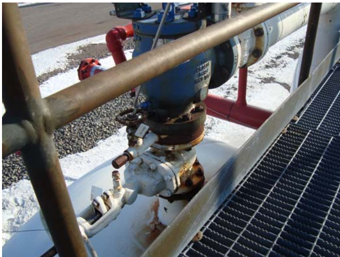
Photo 31 – Nozzle N7, slight coating breakdown, studs and nuts CAT III
