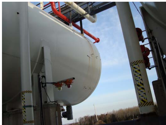
Photo 10 – General condition of paint coating, photo of the East side shell, taken facing North. Small isolated patches of coating breakdown along upper section of sidewall, largest patch measuring approx 150mm x 150mm
