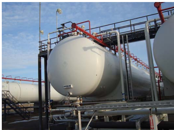
Photo 7 – General condition of paint coating, photo of the East side shell, taken facing North. Small isolated patches of coating coating breakdown along upper section of sidewall, largest patch measuring approx 150mm x 150mm
