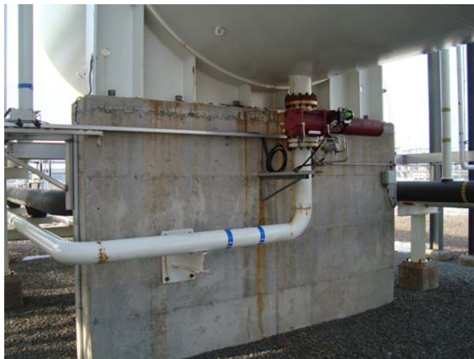
Photo 4 – North face of South vessel support, coating breakdown on lower flange and on edges of vertical stiffeners
