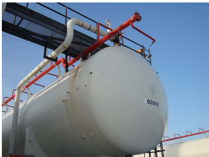
Photo 11 – North dome end, one isolated patch of coating breakdown, slight corrosion evident, and water staining coming from vessel walkway support
