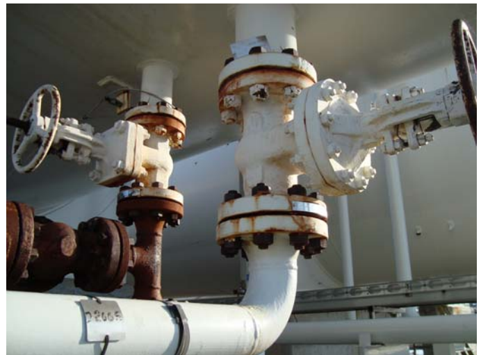
Photo 20 – Nozzles N3B &amp; N4B, coating breakdown and slight corrosion. Studs and nuts CAT III
