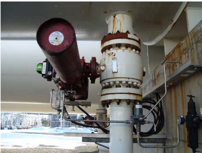
Photo 23 – Nozzle N2 with light to moderate corrosion and coating breakdown. Studs and nuts CAT III
