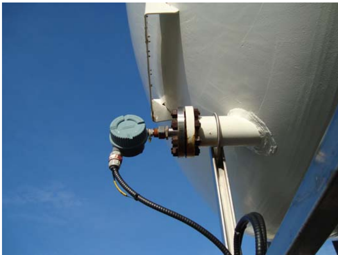
Photo 19 – Nozzle N6, generally in good condition. Stud bolts and nuts CAT III
