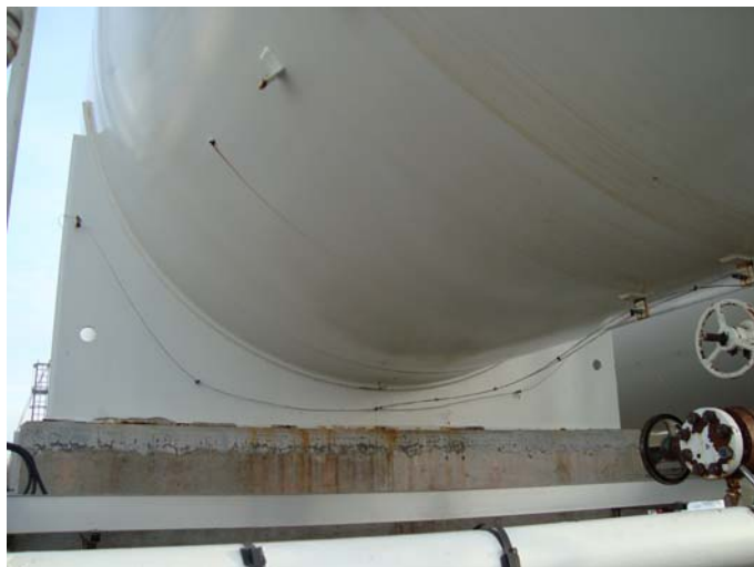
Photo 3 – South face of South vessel support, in good condition. Coating breakdown only on lower flange
