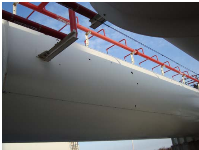
Photo 9 – General condition of paint coating, photo of the East side shell, taken facing North. Small isolated patches of coating breakdown along upper section of sidewall, largest patch measuring approx 150mm x 150mm
