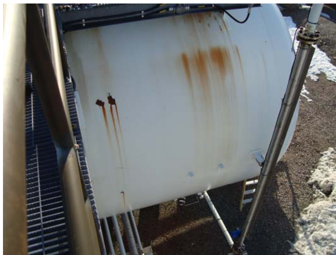
Photo 28 – West side wall next to South dome end showing discoloration of vessel and coating breakdown
