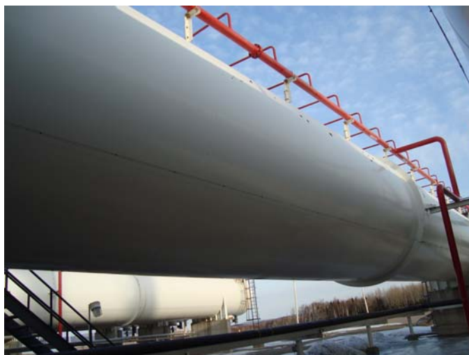
Photo 8 –General condition of paint coating, photo of the East side shell, taken facing North. Small isolated patches of coating coating breakdown along upper section of sidewall, largest patch measuring approx 150mm x 150mm
