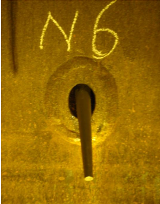
Photo 13 – Nozzle N6 – Thermowell south end.
