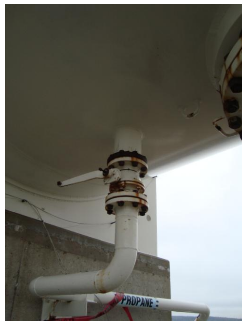
Photo 4 – (N5) Studs and nuts CAT II, 100% coating breakdown with surface corrosion on flange
