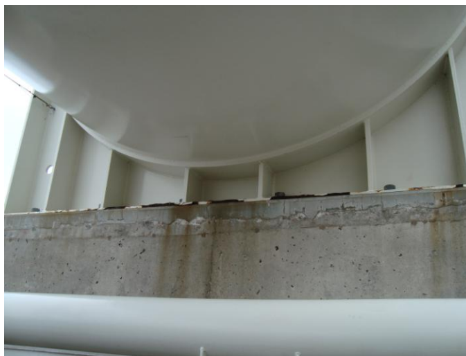
Photo 6 – Coating breakdown with surface corrosion occurring at foot of saddle support leg. This appears to be common of all propane storage vessels in this location
