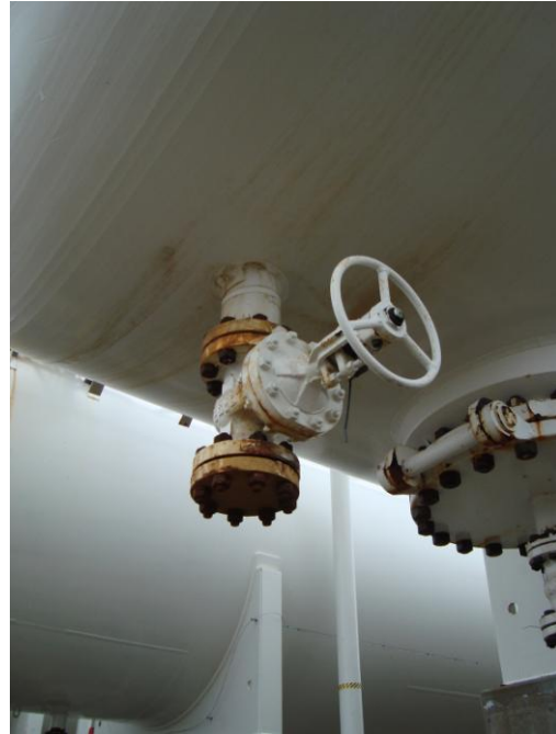
Photo 2 – (N10) Studs and nuts CAT II, 20% coating breakdown with surface corrosion on flange
