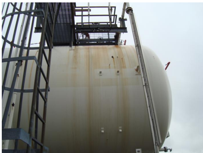
Photo 11 – View of South-West end of vessel. Isolated areas of coating breakdown with surface corrosion. There does not appear to be any significant material loss
