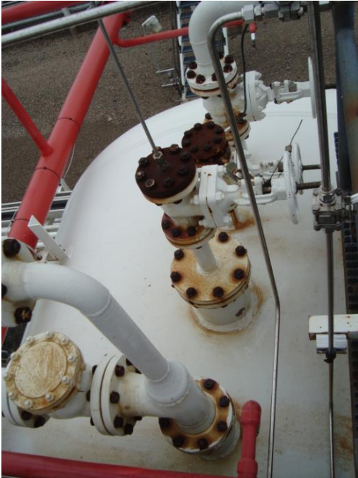
Photo 17 – (N1, N8, N4A, N3A) Studs and nuts CAT II. 100% coating breakdown with surface corrosion of blank flanges. Small amount of coating breakdown with surface corrosion occurring on nozzles
