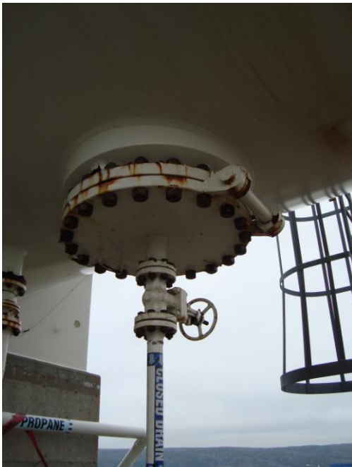
Photo 3 – (M) Studs and nuts CAT II, 20% coating breakdown with surface corrosion on flange
