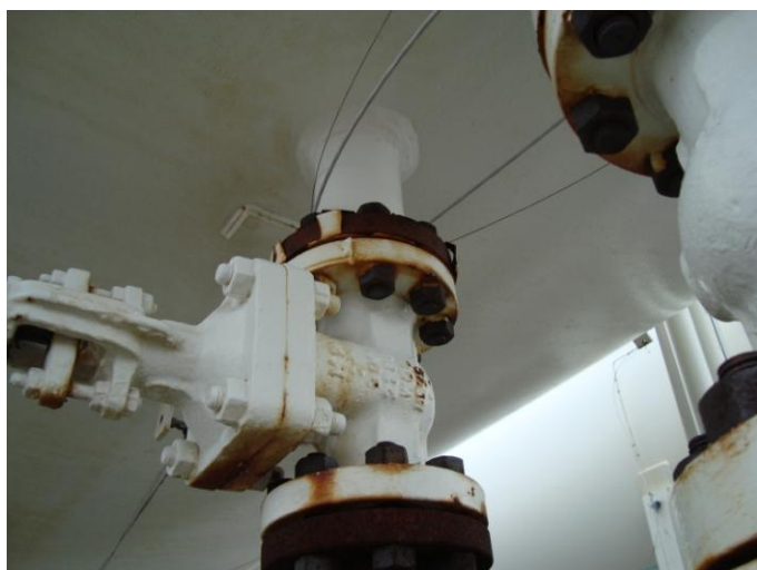
Photo 15 – (N4B) 60% coating breakdown with surface corrosion on flange. Studs and nuts CAT II
