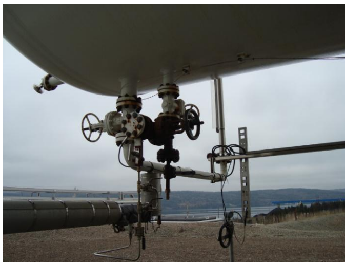
Photo 10 – (N3B, N4B) Trim attached to N4B has 100% coating breakdown with surface corrosion. 60% coating breakdown with surface corrosion on flanges, studs and nuts CAT II
