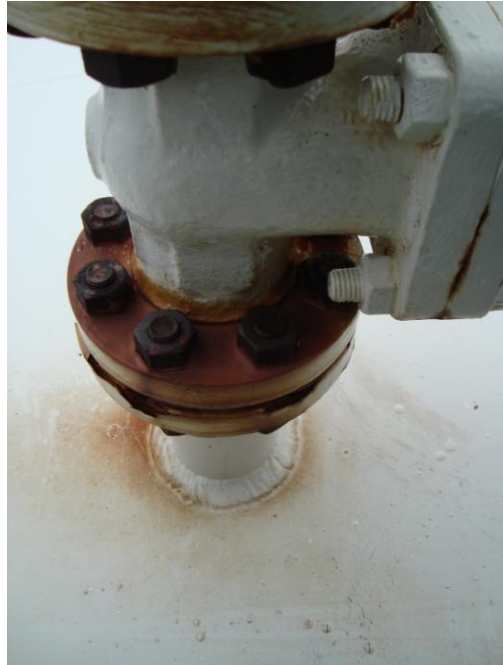
Photo 18 – (N9) Studs and nuts CAT II. 60% coating breakdown with surface corrosion occurring on flanges
