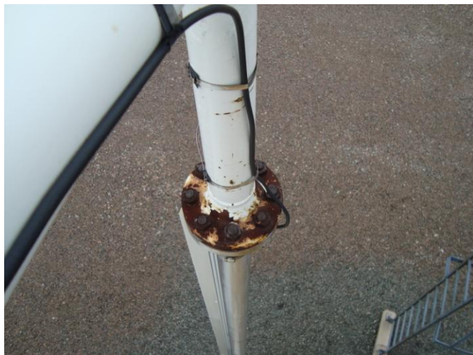
Photo 21 – Vessel level gauge as viewed from above. Note: Use of dissimilar metals. 80% coating breakdown with surface corrosion on flange. Studs and nuts CAT II
