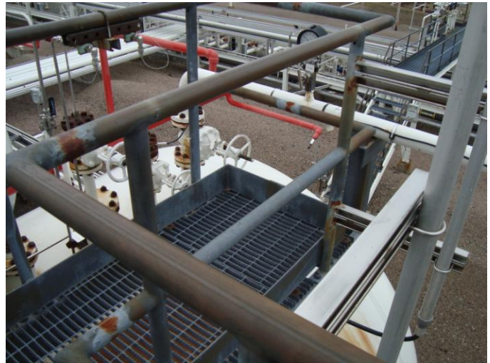
Photo 20 – Isolated areas of coating breakdown with surface occurring on access way
