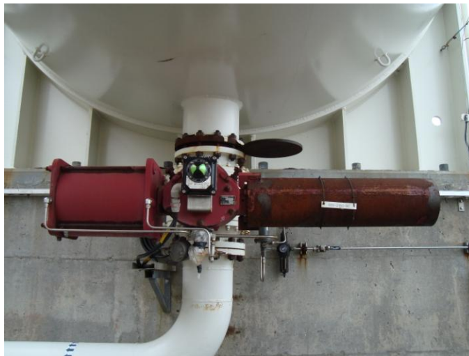
Photo 8 – (SDV2100) 50% coating breakdown with surface corrosion of valve. 90% coating breakdown with surface corrosion on flange of N2. Studs and nuts CAT II
