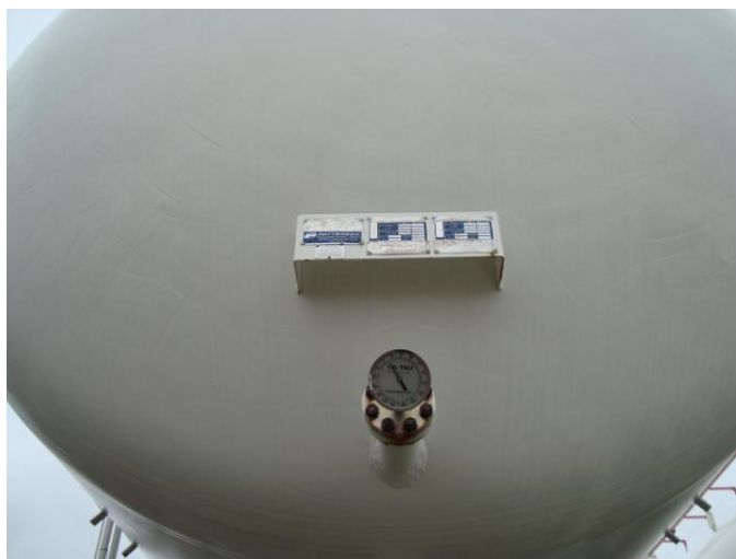
Photo 12 – (N6) Note: Use of dissimilar metals. Gauge in good condition, studs and nuts CAT II. Note: Grind marks/scores on dome end of vessel
