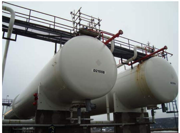
Photo 24 – General good condition of North dome end, photo taken facing South
