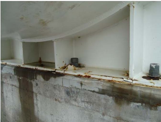
Photo 3 – Steel to concrete connection, coating breakdown mainly on edges
