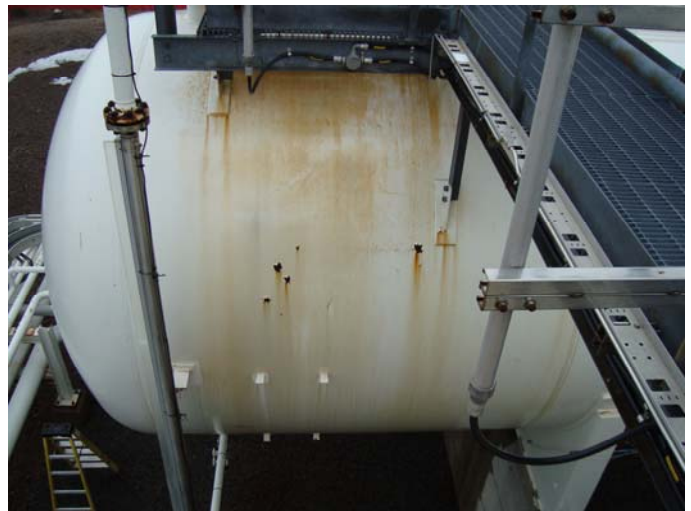
Photo 28 – Showing 4 small isolated patches of coating breakdown and light corrosion on the upper South-East side shell Dome end
