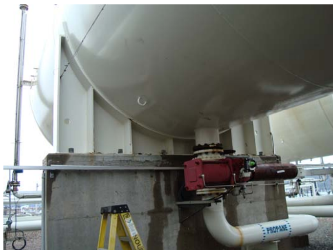
Photo 5 – North face of South vessel support, paint coating in good condition. Coating breakdown on lower flange mainly
