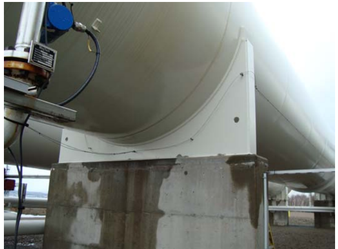
Photo 4 – South face of South vessel support, paint in good condition
