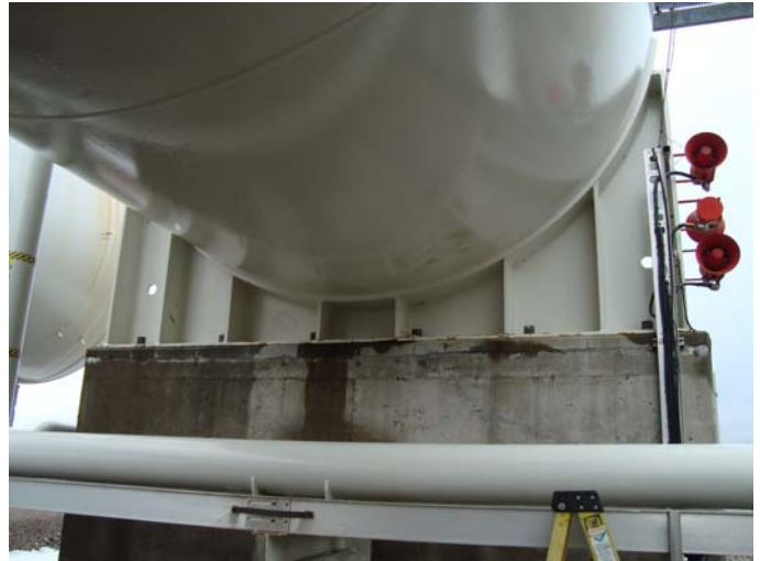
Photo 2 – Showing South face of North vessel support, coating breakdown and corrosion only on lower flange connection to concrete
