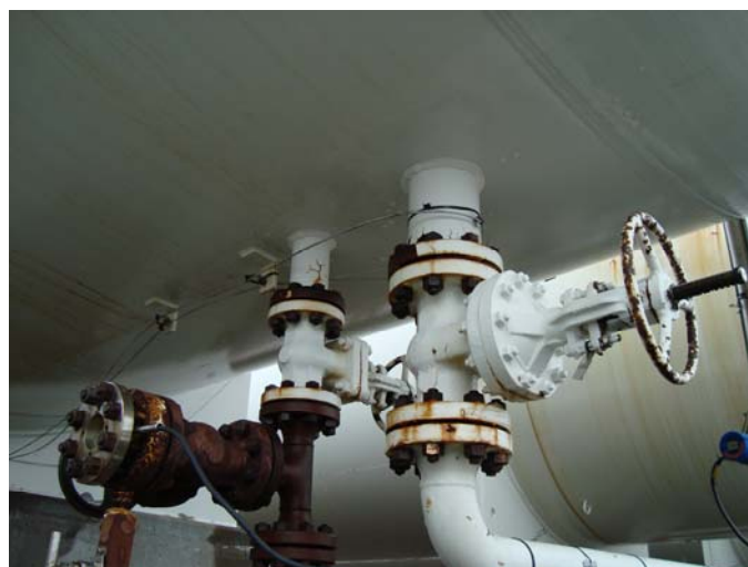
Photo 16 – Nozzles N3B &amp; N4B, coating breakdown and light corrosion located on nozzle body and flange, studs and nuts CAT III
