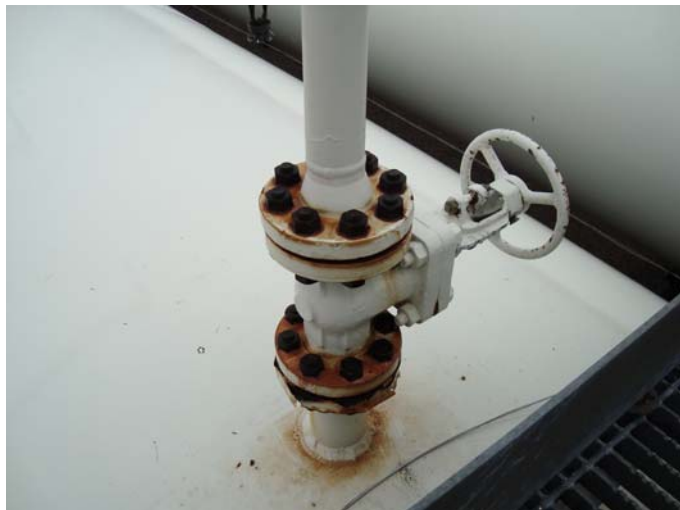
Photo 31 – Nozzle N9, coating breakdown on flange connection, only studs and nuts have lost paint coating but are still in good condition, CAT III
