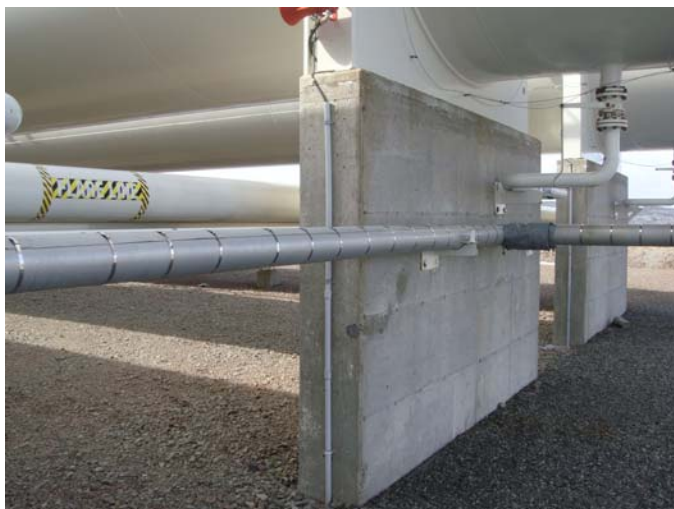
Photo 8 – Earthing strap and connections on North vessel support
