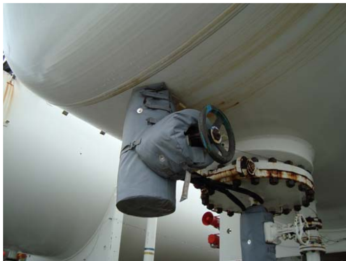
Photo 20 – N10, insulation bag in good condition, studs and nut CAT III
