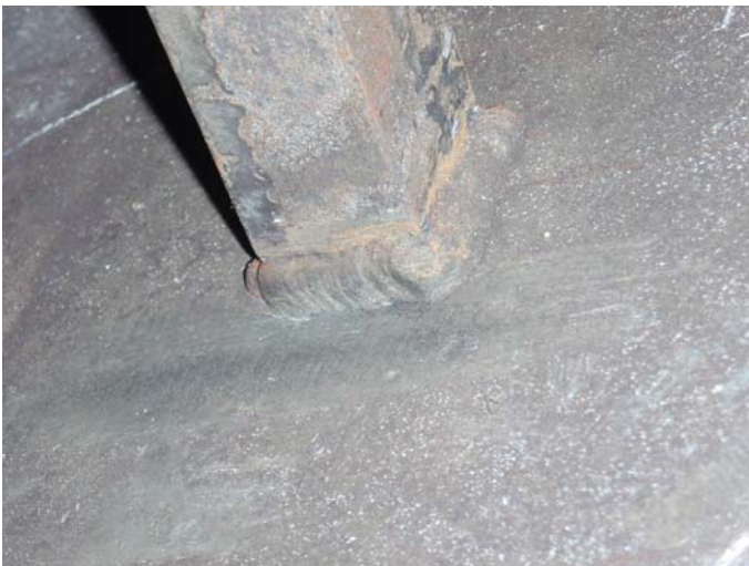
Photo 11 – Close view of the weld for Vortex breaker to shell
