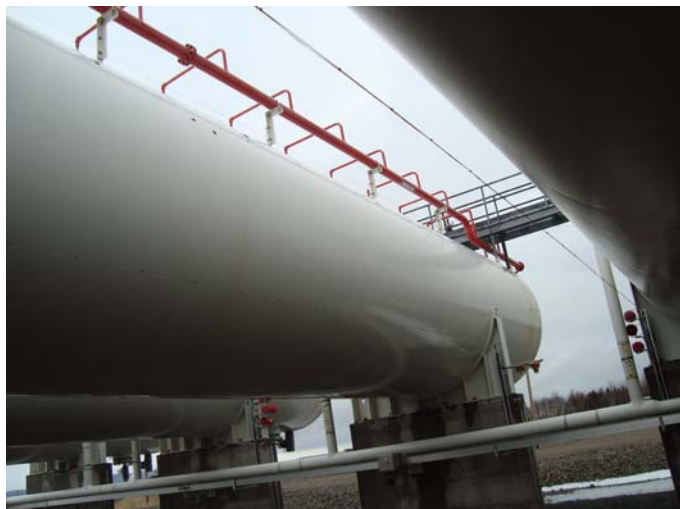
Photo 23 – General condition of East side shell, only a few small isolated patches of coating breakdown and light corrosion located on the upper section of shell
