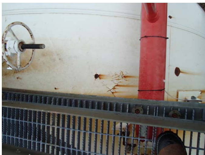
Photo 36 – Coating breakdown and light corrosion on top of North dome, East side
