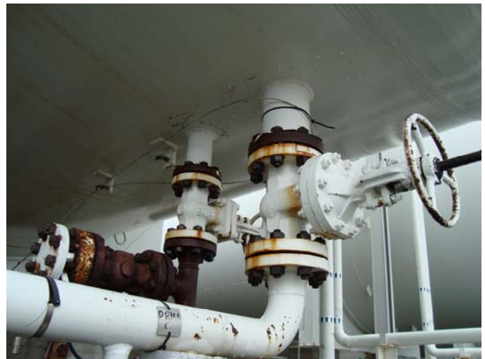
Photo 16 – Nozzles N3B &amp; N4B, coating breakdown and light corrosion located only on flange connection, studs and nuts CAT III
