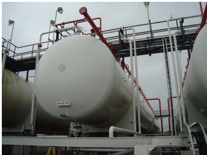
Photo 21 – General condition of East side shell, only a few small isolated patches of coating breakdown and light corrosion located on the upper section of shell
