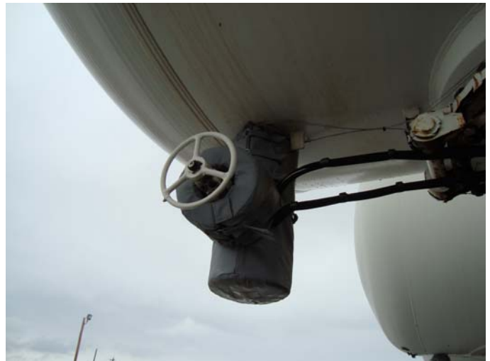
Photo 20 – N10, insulation bag in good condition, studs and nuts CAT III
