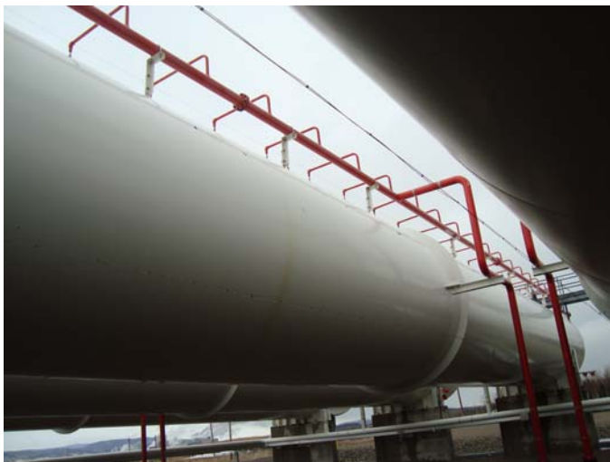
Photo 22 – General condition of East side shell, only a few small isolated patches of coating breakdown and light corrosion located on the upper section of shell
