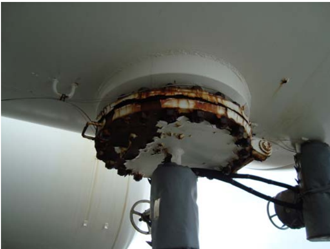
Photo 19 – Manhole, coating breakdown on flanges only. Studs and nuts uncoated, CAT III
