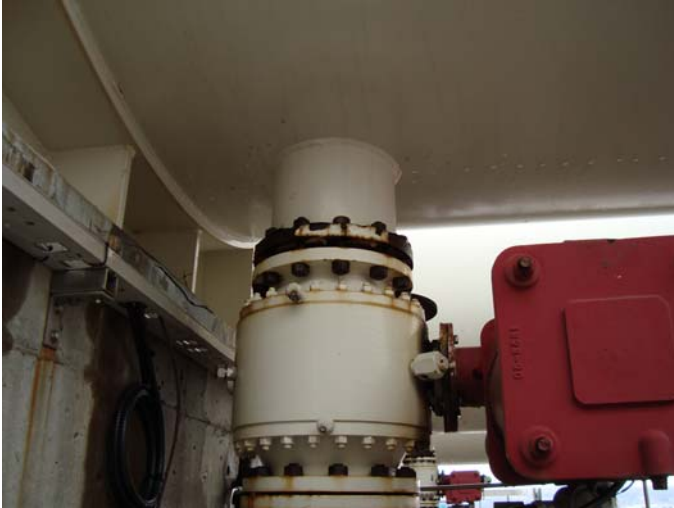
Photo 17 – Nozzle N2, coating breakdown only on flange connection. Studs and nuts uncoated but in good condition, CAT III
