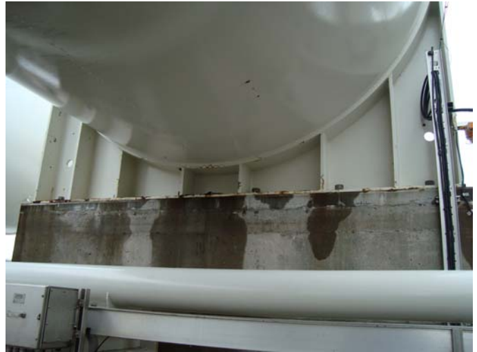
Photo 2 – South face of North vessel support, coating breakdown and corrosion only on lower flange connection to concrete
