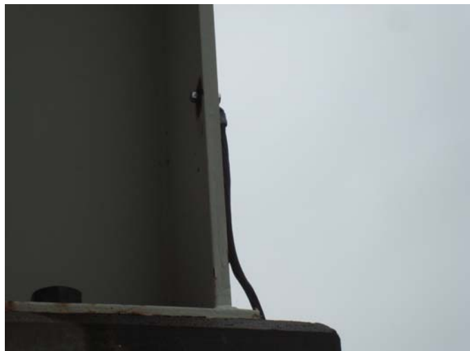
Photo 7 – Earth strap connections to be in good condition
