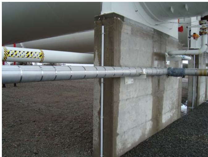
Photo 8 – Earth strap connections to be in good condition
