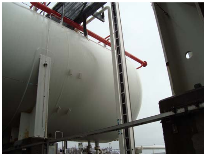
Photo 23 – West side shell of vessel, in good condition, photo taken facing South
