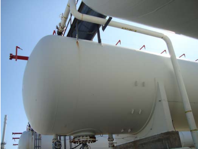
Photo 25 – General good condition of West side shell only one patch of coating breakdown shown, photo taken facing South
