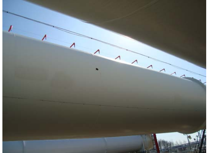
Photo 26 – General good condition of West side shell only one patch of coating breakdown shown, photo taken facing South
