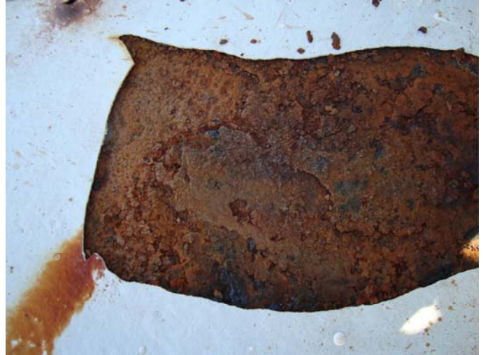
Photo 38 – Showing patch next to N7 largest area of coating breakdown found so far approx 200mm x 150mm light to moderate corrosion. The corrosion will be removed and a UT scan will be carried out and noted in the UT report
