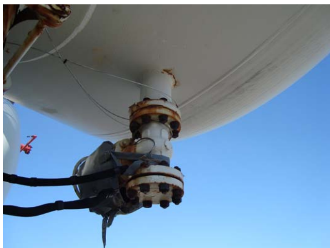
Photo 19 – Nozzle N10, slight coating breakdown on weld connection and flange no insulation bag present
