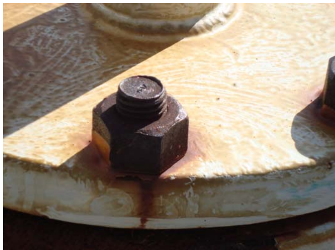
Photo 31 – Close-up of nozzle N8 showing a good example of the condition of the nuts and bolts on this vessel
