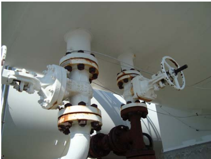
Photo 15 – Nozzles N3B &amp; N4B in good condition, studs and nuts CAT III
