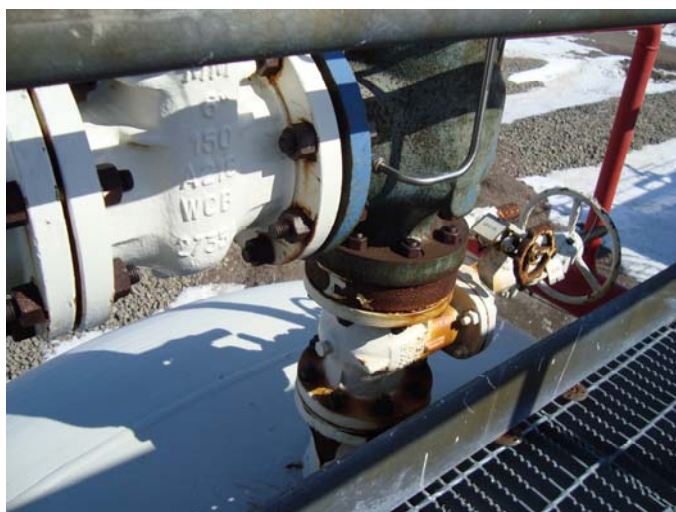
Photo 36 – Nozzle N7 PSV, coating breakdown around nozzle studs and nuts CAT III
