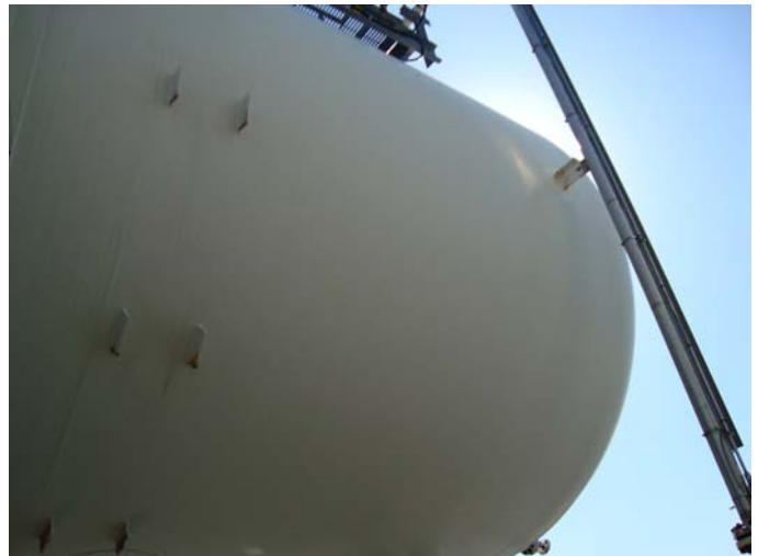
Photo 28 – General good condition of West side shell only one patch of coating breakdown shown, photo taken facing South
