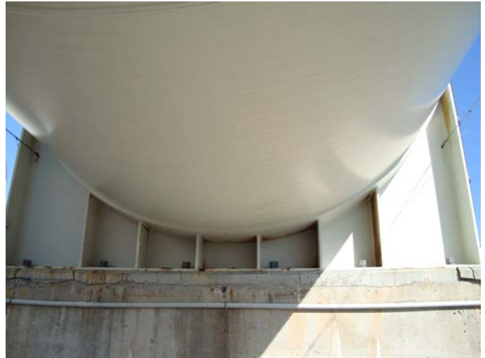
Photo 2 – South face on North vessel support coating breakdown on concrete connection, weld connections on vertical stiffeners starting to break down
