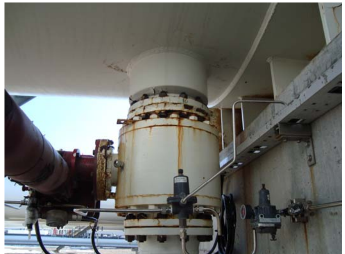
Photo 16 – Nozzle N2, slight coating coating breakdown on nozzle, studs and nuts CAT III
