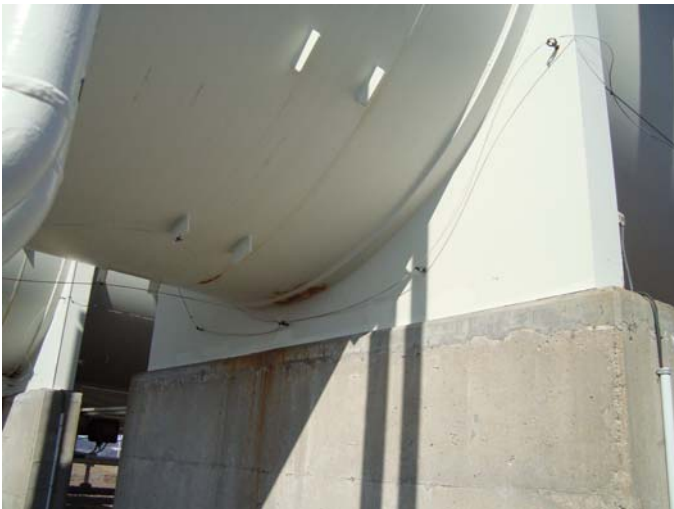
Photo 3 – South vessel support south face slight coating breakdown on cradle and vessel
