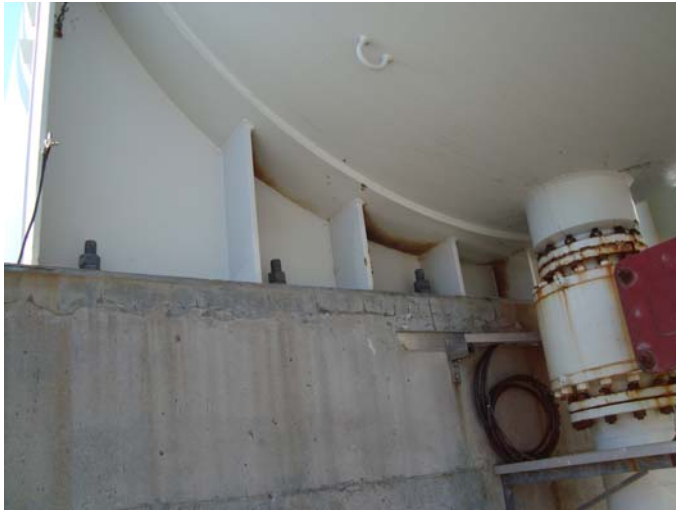
Photo 5 – North face of South vessel support slight coating breakdown on concrete connection and coating breakdown on cradle
