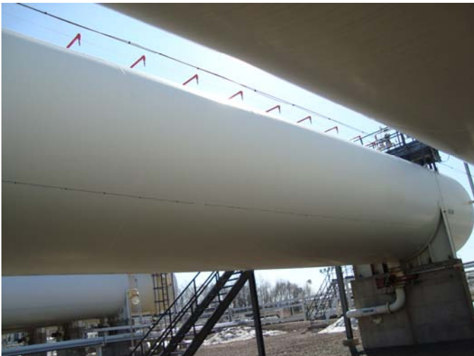
Photo 27 – General good condition of West side shell only one patch of coating breakdown shown, photo taken facing South
