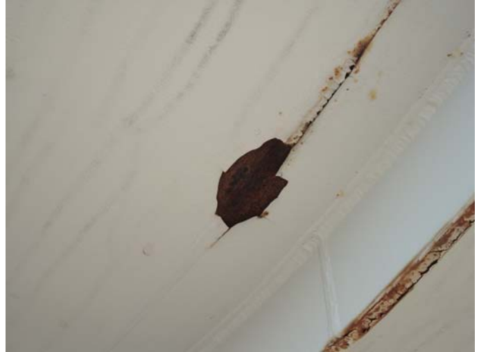
Photo 22 – Showing general condition of east side shell. Taken facing North, showing one isolated patch located in the mid bottom section on weld seam approx 100mm x 100mm
