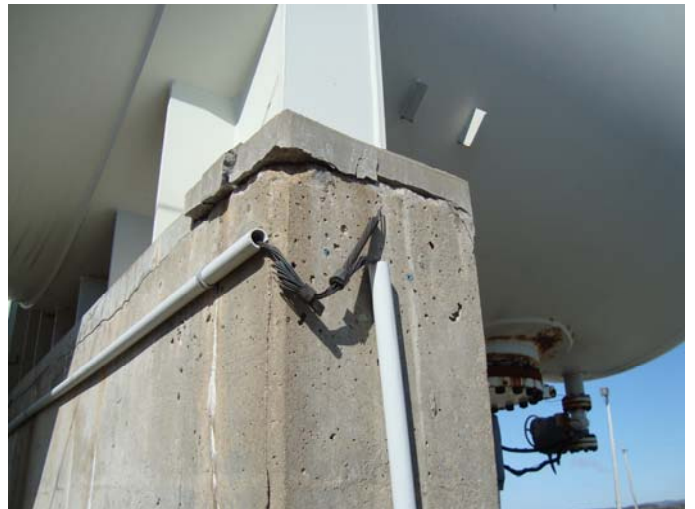
Photo 8 – Earthing strap Joint on North vessel support, also showing horizontal crack in concrete support
