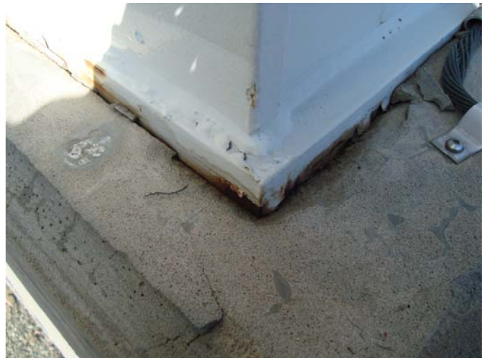
Photo 4 – South vessel support South-East corner water damage to concrete
