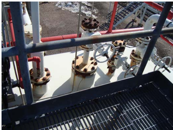
Photo 30 – Nozzels located at South end top N3A, N4A, N8 & N1, showing general condition all studs and nuts at this location are in good condition, CAT III
