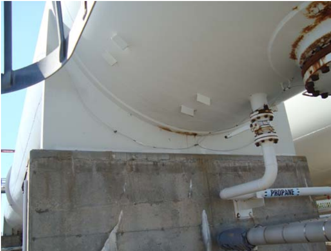
Photo 1 – North face on North vessel support coating breakdown on steel to concrete connection, also coating breakdown on weld connection to vessel
