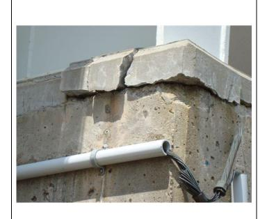
Photo 9 – North Foundation support – crack in concrete
