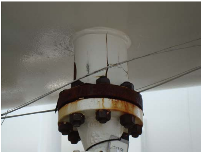
Photo 19 – Flange in fair condition with 100% coating breakdown, no notable substrate loss
