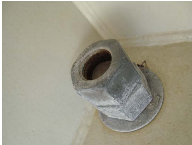
Photo 10 – General condition of studs and nuts, good condition. North end structural support bolts are correctly positioned with expansion-purpose gap between bolt and vessel. South end structural support bolts are lacking in thread protrusion up to 20mm
