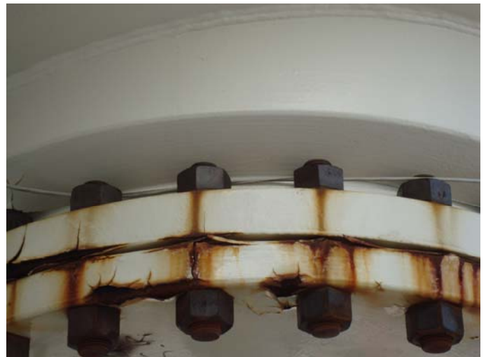
Photo 20 – Flange in fair condition with delamination of coating, no notable substrate loss
