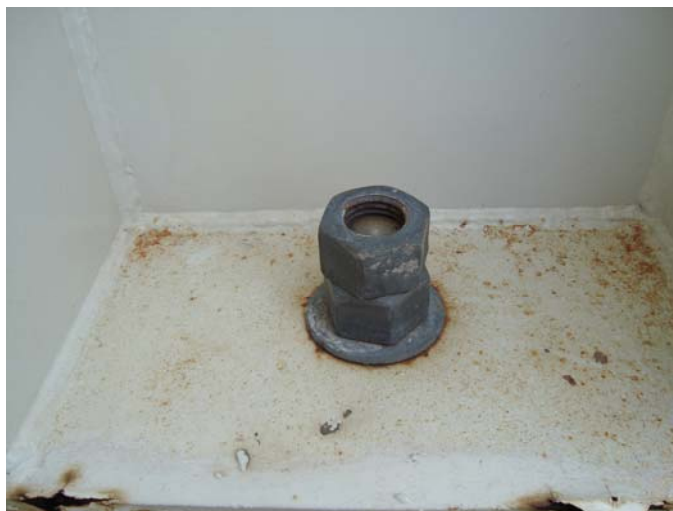
Photo 8 –General condition of studs and nuts, good condition. North end structural support bolts are correctly positioned with expansion-purpose gap between bolt and vessel. South end structural support bolts are lacking in thread protrusion up to 20mm
