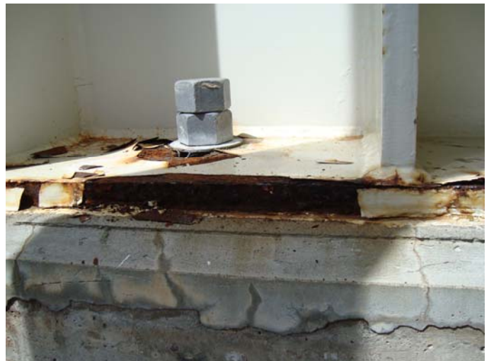
Photo 4 –General condition of studs and nuts, good condition. North end structural support bolts are correctly positioned with expansion-purpose gap between bolt and vessel. South end structural support bolts are lacking in thread protrusion up to 20mm
