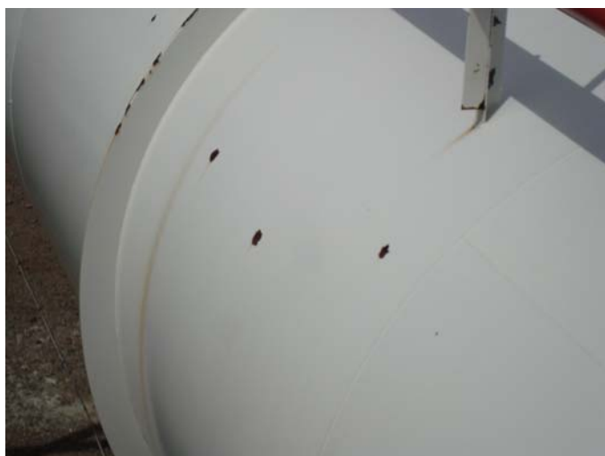
Photo 27 – Isolated areas of coating breakdown on shell, no notable substrate loss, grade 6S-7S
