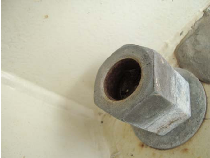
Photo 13 – General condition of studs and nuts, good condition. North end structural support bolts are correctly positioned with expansion-purpose gap between bolt and vessel. South end structural support bolts are lacking in thread protrusion up to 20mm
