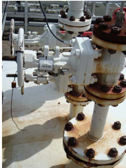
Photo 30 – Flange in fair condition with 100% coating breakdown, no notable substrate loss
