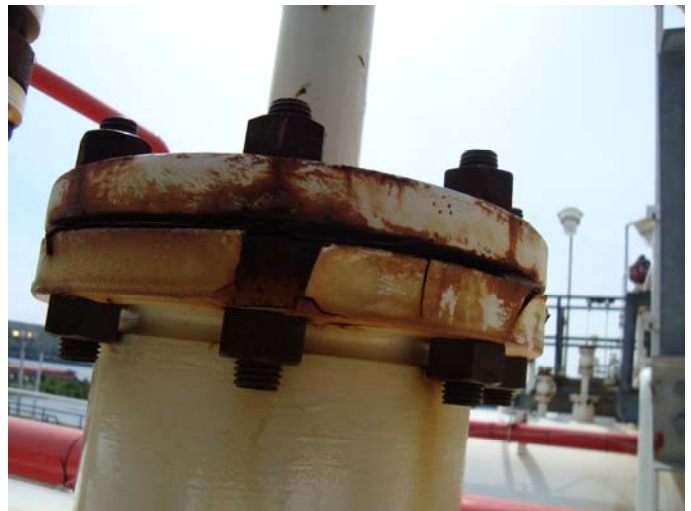
Photo 24 – Flange in fair condition with coating breakdown &amp; delamination, no notable substrate loss
