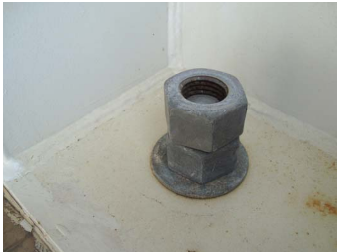
Photo 9 – General condition of studs and nuts, good condition. North end structural support bolts are correctly positioned with expansion-purpose gap between bolt and vessel. South end structural support bolts are lacking in thread protrusion up to 20mm
