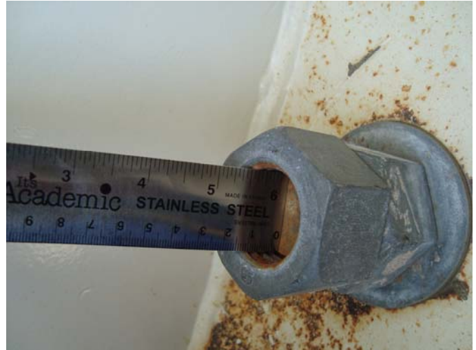
Photo 14 – General condition of studs and nuts, good condition. North end structural support bolts are correctly positioned with expansion-purpose gap between bolt and vessel. South end structural support bolts are lacking in thread protrusion up to 20mm
