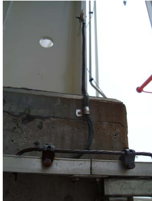
Photo 18 – Grounding cable intact and in good condition
