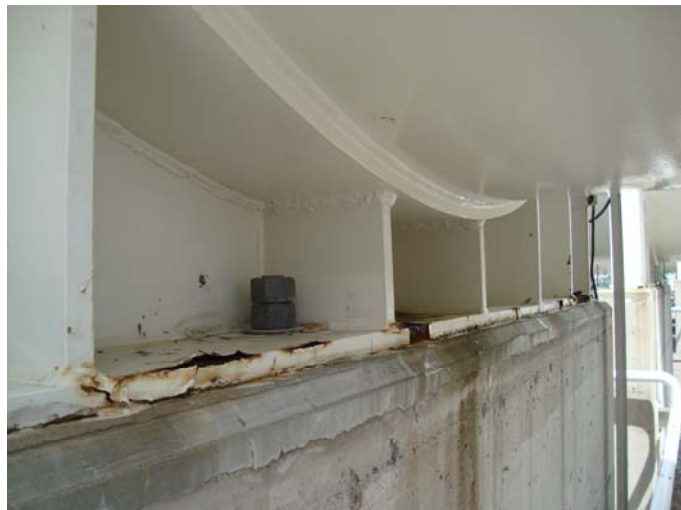
Photo 5 – General condition of studs and nuts, good condition. North end structural support bolts are correctly positioned with expansion-purpose gap between bolt and vessel. South end structural support bolts are lacking in thread protrusion up to 20mm
