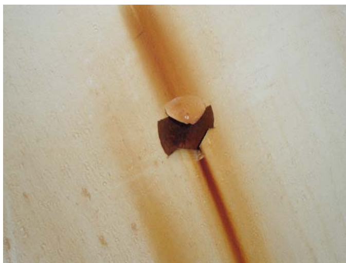
Photo 28 – Isolated areas of coating breakdown on shell, no notable substrate loss, grade 6S-7S
