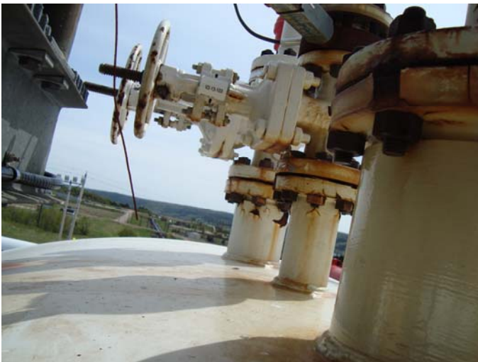
Photo 23 – Flange in fair condition with partial coating breakdown &amp; delamination, no notable substrate loss
