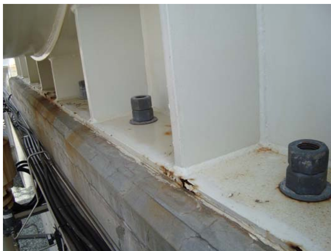
Photo 12 – General condition of studs and nuts, good condition. North end structural support bolts are correctly positioned with expansion-purpose gap between bolt and vessel. South end structural support bolts are lacking in thread protrusion up to 20mm
