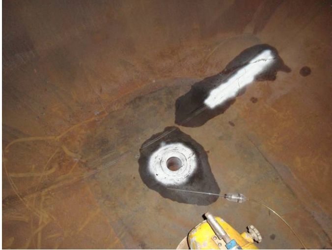
Photo 15 – Looking down at nozzle N10-3” from interior of vessel
