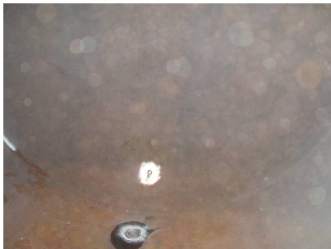
Photo 3 – Looking down at nozzle N6-2” thermowell on South head
