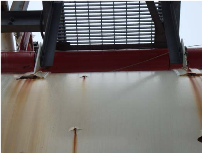
Photo 17 – Coating breakdown and rust staining propagating from re-enforcement plates of access way supports
