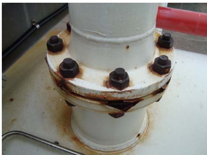
Photo 23 – (N1) Studs and nuts CAT II, 30% coating breakdown with surface corrosion on flange
