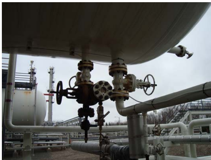
Photo 13 – (N4B) 40% coating breakdown with surface corrosion occurring on flange. Studs and nuts CAT II, 100% coating breakdown with surface corrosion of vessel trim attached
