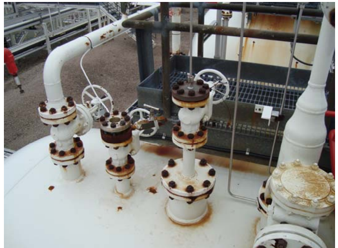
Photo 20 – (N3A, N4A, N8) Studs and nuts CAT II, coating breakdown with surface corrosion occurring on trim
