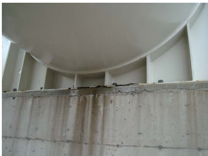
Photo 7 – Coating breakdown with surface corrosion occurring at foot of saddle support. This is a general occurrence of all the propane storage vessels
