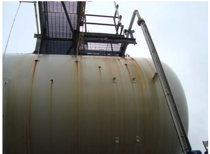
Photo 12 – Areas of coating breakdown with surface corrosion on South-West end of vessel. Corrosion appears to be light
