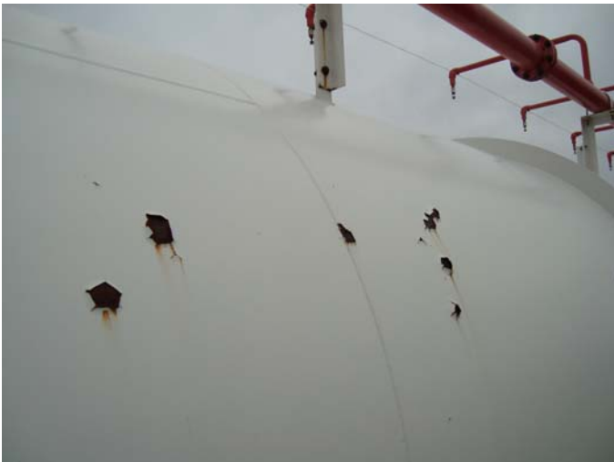
Photo 19 – Areas of coating breakdown with surface corrosion occurring on East side of vessel
