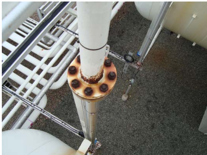
Photo 27 – Condition of vessel level gauge as viewed from above. Studs and nuts CAT II. Note: The use of similar metals
