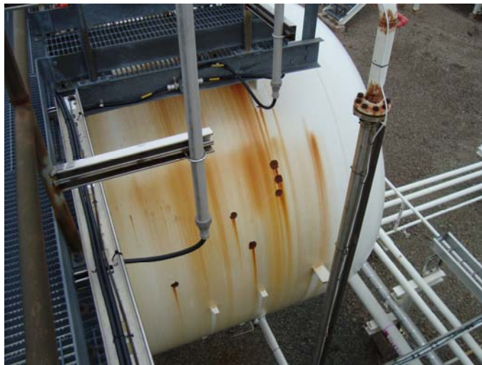
Photo 26 – Coating breakdown with surface corrosion occurring on South-West end of vessel. Rust staining also appears to be stemming from light coating breakdown with surface corrosion on access way
