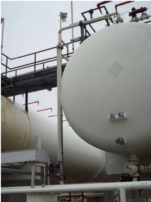
Photo 29 – View of vessel level gauge, in good condition. Note: The use of dissimilar metals
