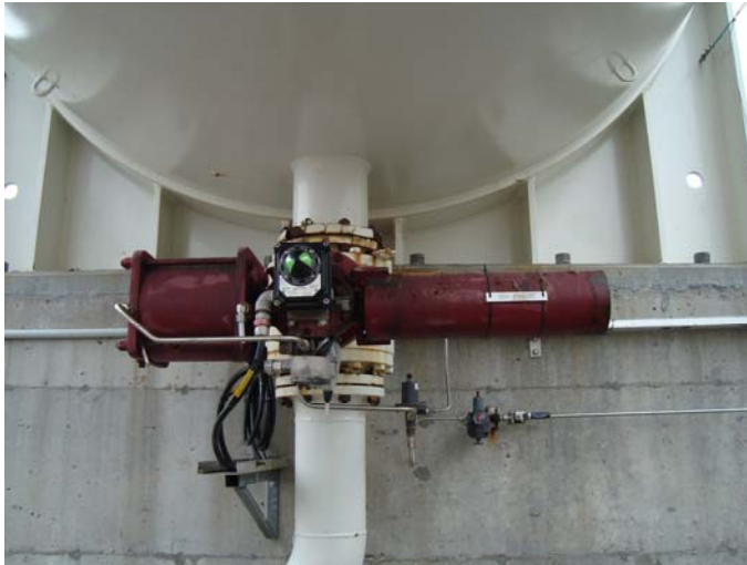
Photo 9 – Condition of SDV2105, 5% coating breakdown with surface corrosion on valve. 10% coating breakdown with surface corrosion occurring on flange of N2
