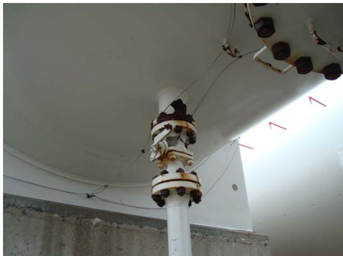
Photo 3 – (N5) 100% coating breakdown with surface corrosion of flange and CAT II studs and nuts. 20% coating breakdown with surface corrosion occurring on nozzle
