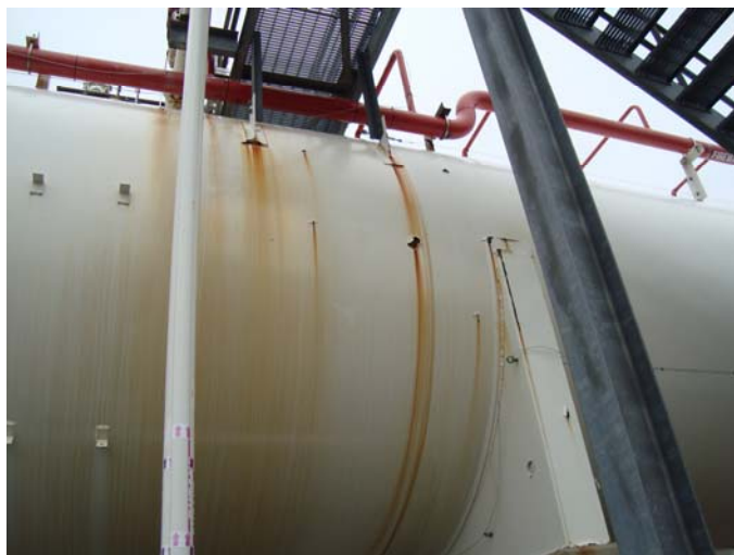
Photo 16 – Areas of coating breakdown with surface corrosion on South-East end of vessel. Corrosion appears to be light. Coating breakdown and rust staining propagating from re-enforcement plates of access way supports
