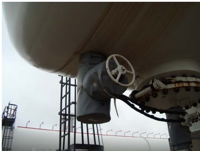
Photo 4 – (N10) Covered by insulation jacket. Heat trace in place, insulation jacket not removed due to proximity of linear heat trace. No CUI appears to be occurring at nozzle. Studs and nuts CAT II
