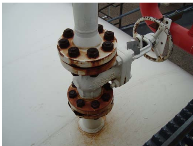
Photo 24 – (N9) Studs and nuts CAT II, 60% coating breakdown with surface corrosion on flange
