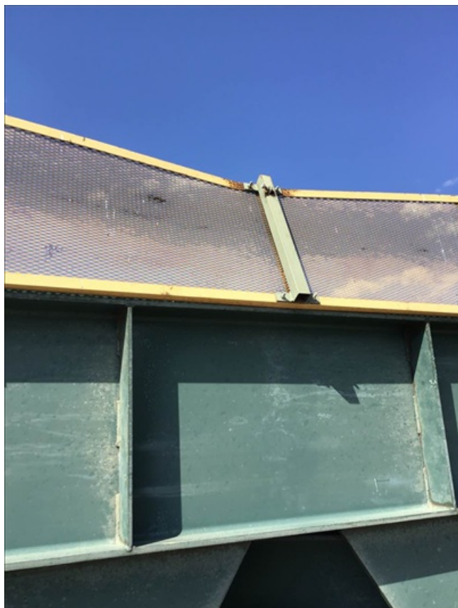
DAMAGED WIND GUARD
